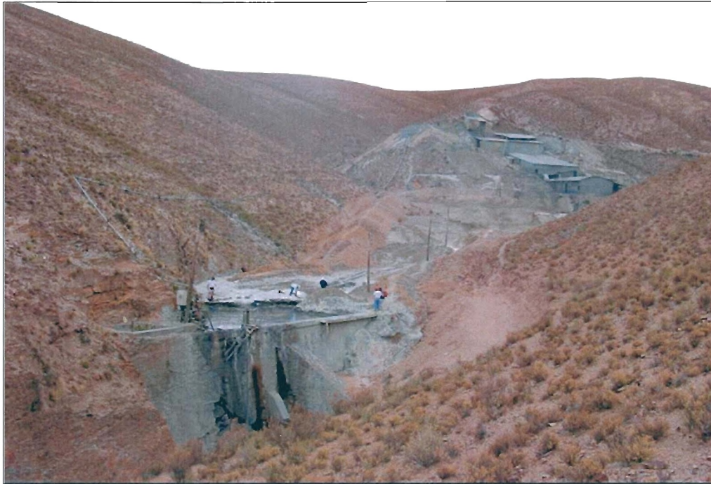
Figure 3. Panoramic view of the Abaróa Valley. A concrete tailings dam traverses the valley in the foreground; dumps and the beneficiation plant are in the background.
