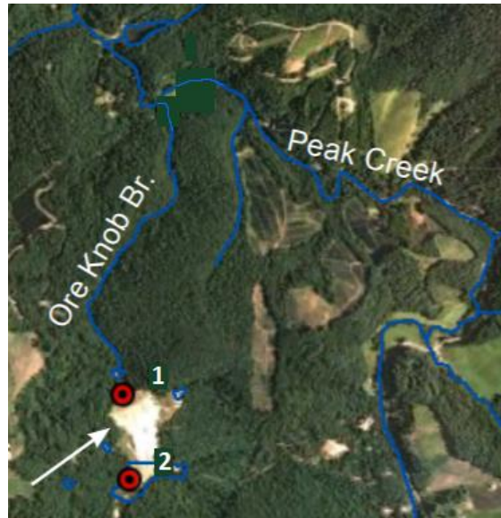
Figure 1. Mine site (white arrow) showing the earthen dam across Ore Knob Branch (1) and the disposed of tailings materials (2) within the Peak Creek Drainage system.
